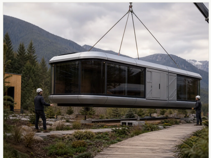
Stage 05: Single-day crane docking on site
